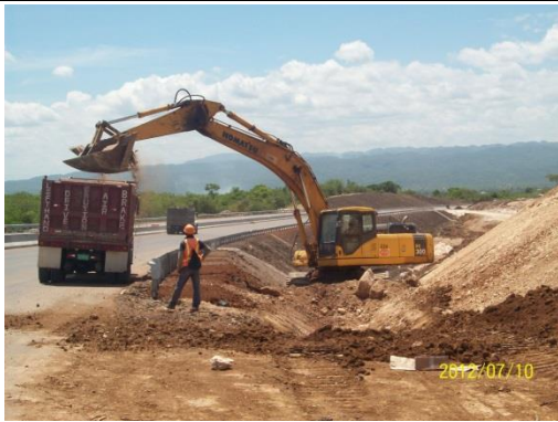
Construction of earth drain along the Sandy Bay Toll Road
