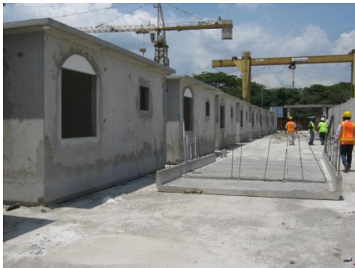
Production of Housing Units at Factory
