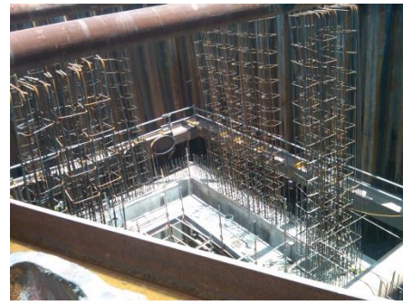
Construction activities on Wet well sump
