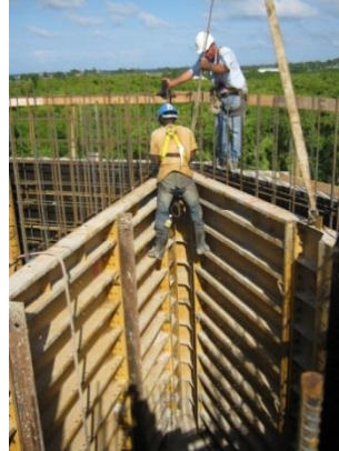
Securing of Formwork for Tower Walls
