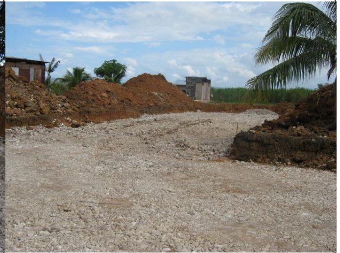
Formation level of roadway being compacted.
