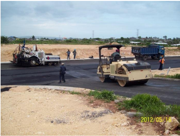
Asphaltic Concrete works
