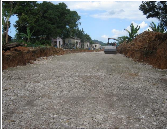
Formation level of roadway being compacted.
