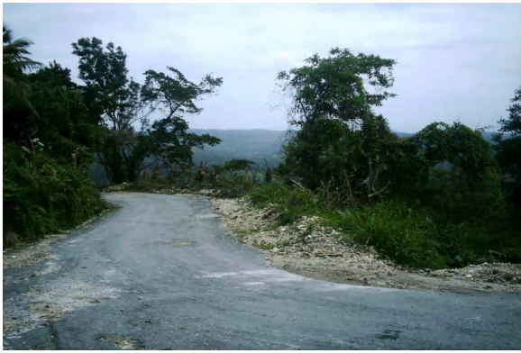
Covered Portion of Pipe Trenches
