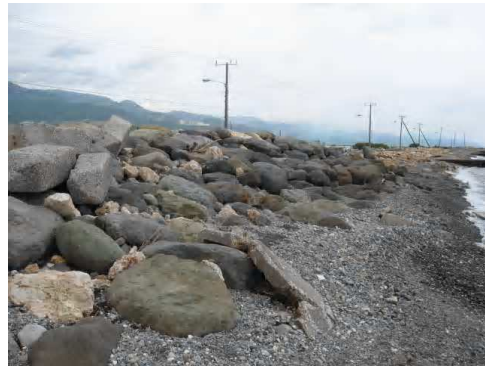
Section of the Revetment
