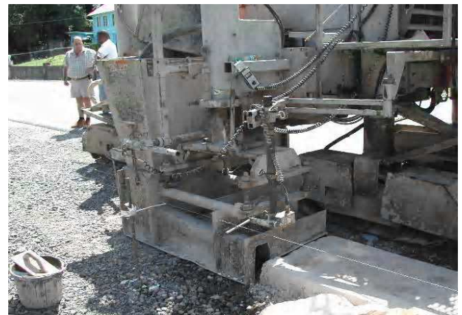
View of concrete drains being constructed in Nov. 2008
