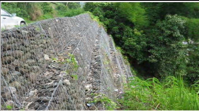
Gabion Basket Retaining Wall
