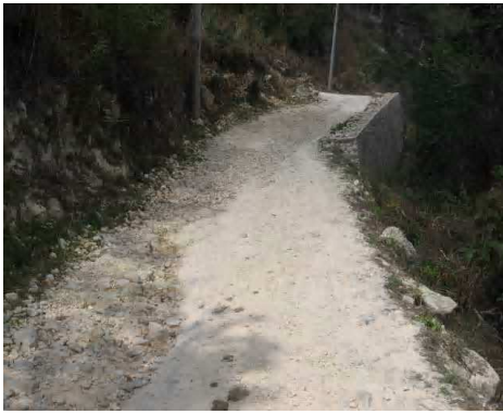
Uncapped Retaining wall
