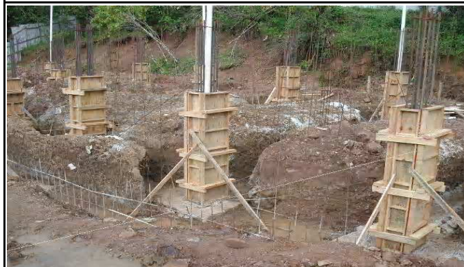
View of Foundation and Concrete Columns
