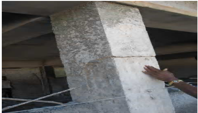
Poor Concreting
