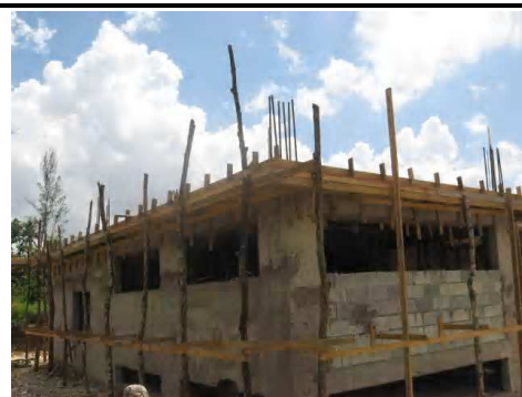
Roof Slab being Prepared for the Pouring of Concrete
