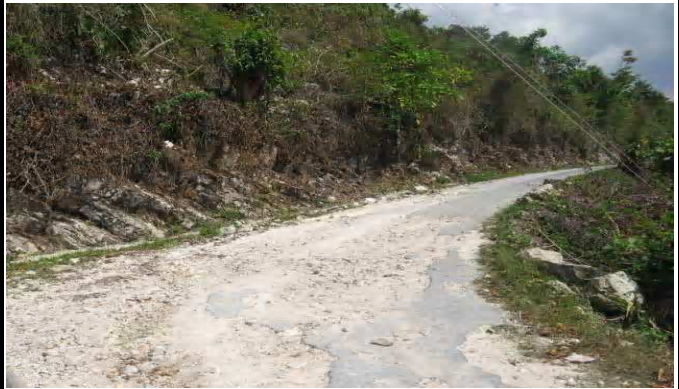
Deterioration of Stabilized Roadway
