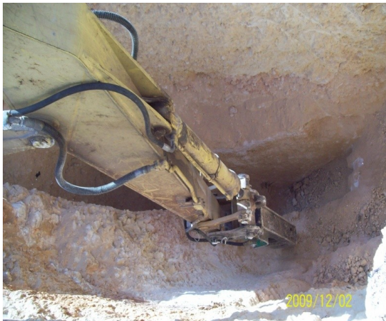
Excavation Works with the Veneer Trencher
