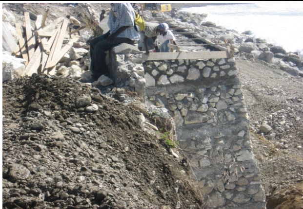
Retaining wall under construction
