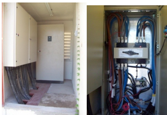
Automatic Transfer Switch Room
