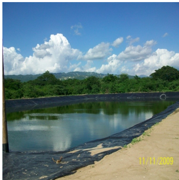
Pond after installation of Polyethylene Liner
