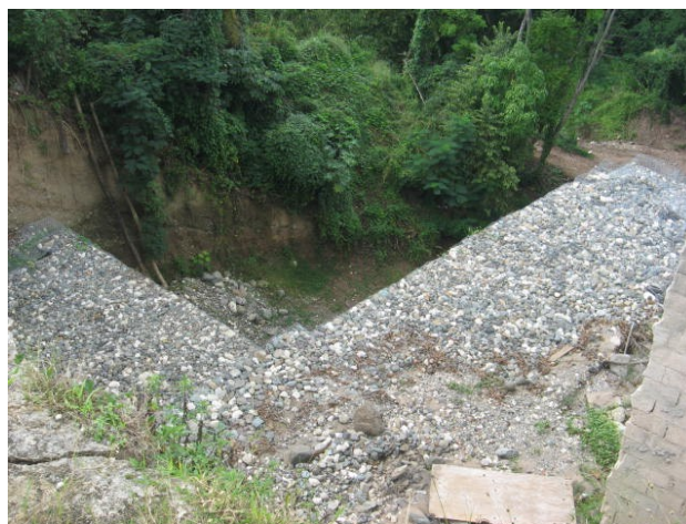
L-Shaped Gabion Wall at Persimmon Ave
