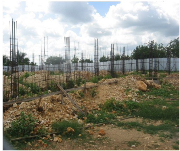
Excavated foundation with steel reinforcement installed
