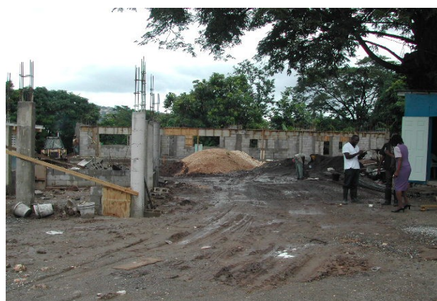
View of ground floor built up to belt beam.
