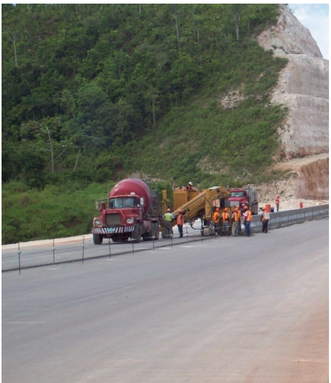
Concrete median being laid
