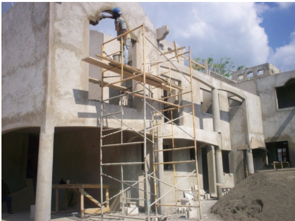
Rendering Work on Unit # 1
