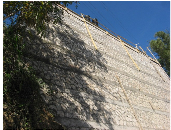
Rubble Retaining Wall Construction in progress
