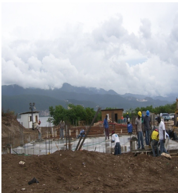
Construction of Raft Foundation in progress
