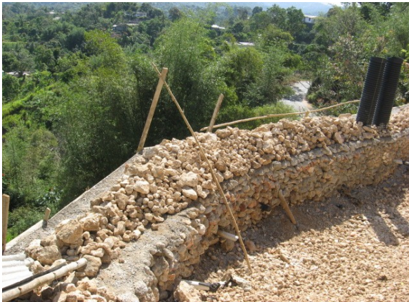
Incomplete Rubble Retaining Wall
