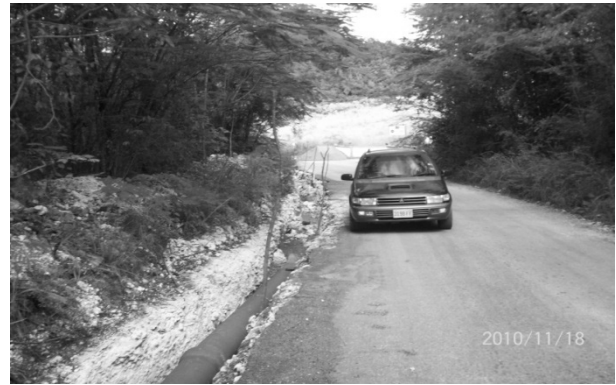
Scouring of Installed Pipe lines Tropical Storm Nicola
