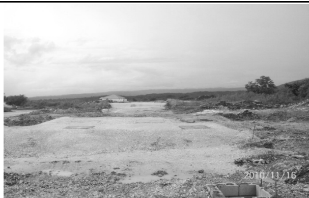
Construction of Marl Pads and Associated Infrastructure for Housing Units
