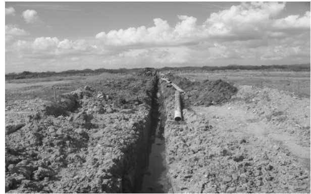
Excavated trench to receive sewage pipes
