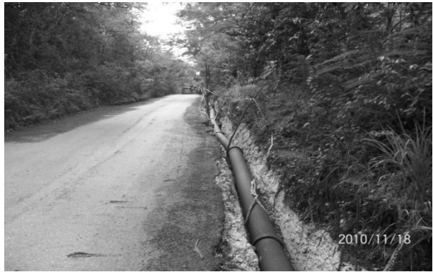
Scouring of Installed Pipe lines due Tropical Storm Nicola
