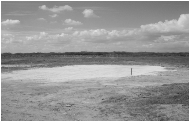
Setting out of pad foundation for Model Unit
