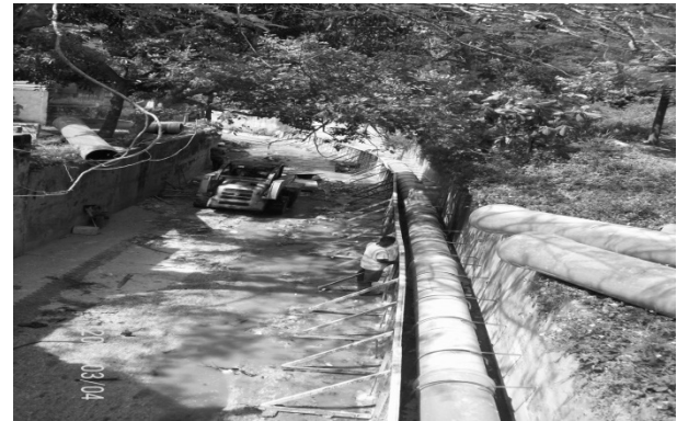
Pipes laid in the North Gully and Installation of form work for casing to protect the pipes.
