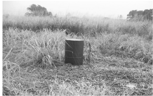
Well Capping at New Forrest
