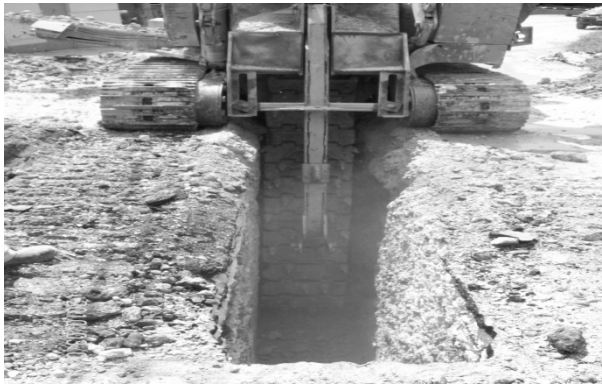
Excavation of trench
