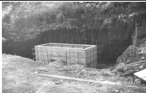
Storm water drainage under construction
